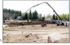
utility connections, footings and foundations. "Right now you can see the footprint of the building," construction manager Doc Smith of EDS Builders said. The pace will continue with the arrival of the pre-cast concrete that will form the walls of the new gymnasium in mid-May and then the 100-foot long roof joists shortly thereafter.
